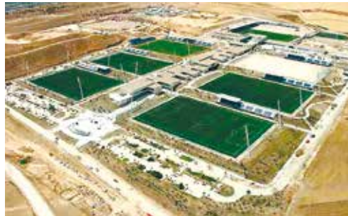
Training centre „REAL MADRID“ (Spain)
