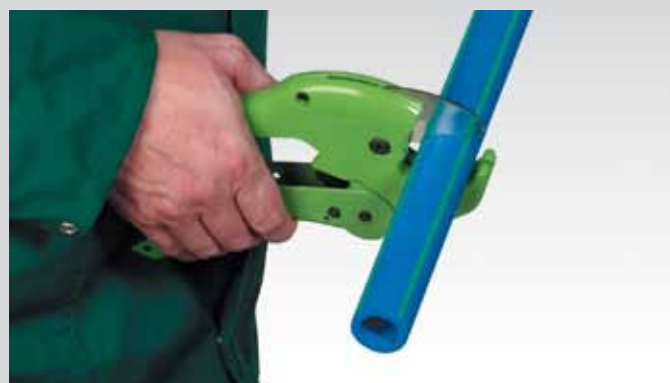
Cutting of the pipe
