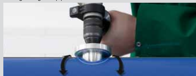
Removal of the oxygen barrier layer from the aquatherm blue pipe of
