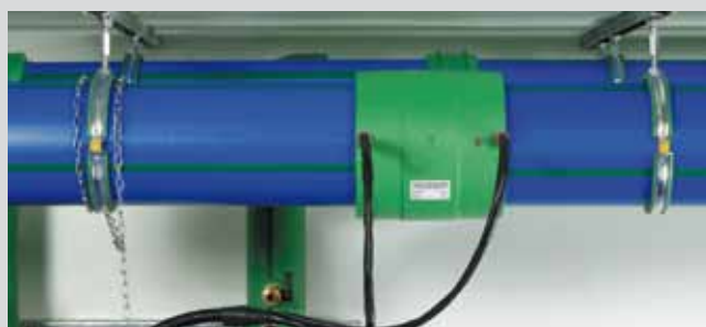
Adjust the socket diameter on the welding device. Start and control welding process. Keep the cooling time. Finished!
