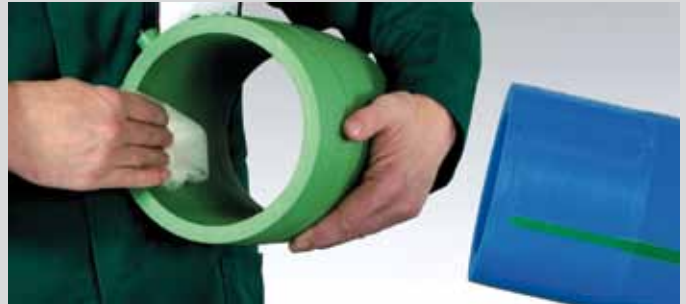
lean the electrofusion socket's inner surface with a lint-free cloth or paper. Remove moisture that may occur immediately before the welding process again.
