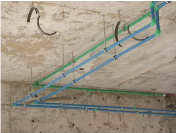
Flex Tower, RAK, UAE
