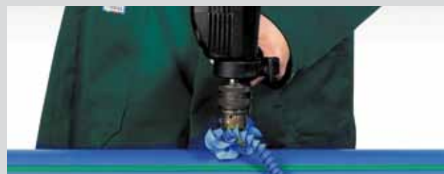
Drilling through the pipe wall
