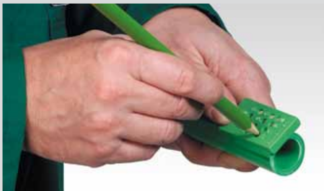
Marking of the welding depth
