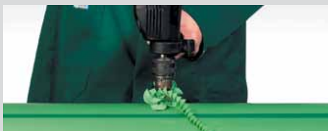
Drilling through the pipe wall
