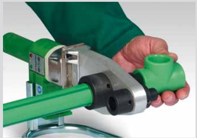
Heating-up of pipe and fitting
