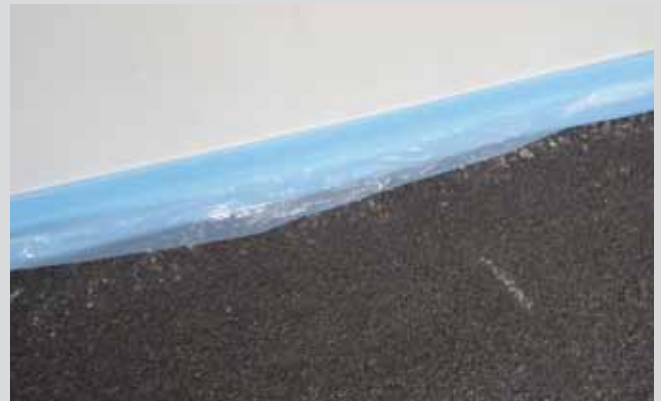
Laying of edge insulation
