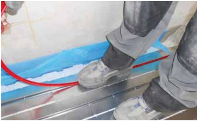
Laying of heating pipes
