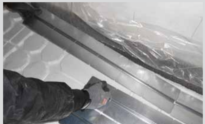
Installation of heat conducting steel sheets
