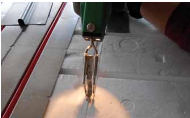
Required extra pipe channels such as connecting pipes are made by filament cutter.
