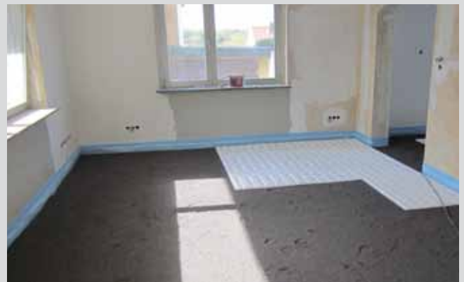
Laying of system element
