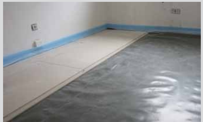
Before installation of the dry elements a release film made of PE is laid.
