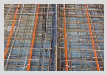
Preparation of construction joints by means of vertically adjustable seam joints
