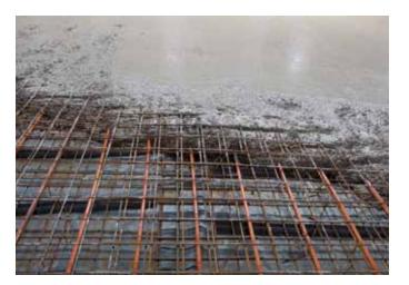
Consistency of the concrete: (WZ-factor 0/5 - 0/6 at minimum 320 kg concrete/m<sup>3</sup>)
