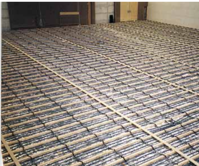
Laying with pipe suspension rail
