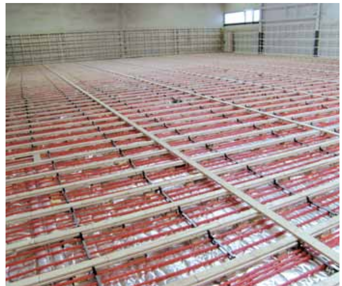
aquatherm orange system sports floor heating system
