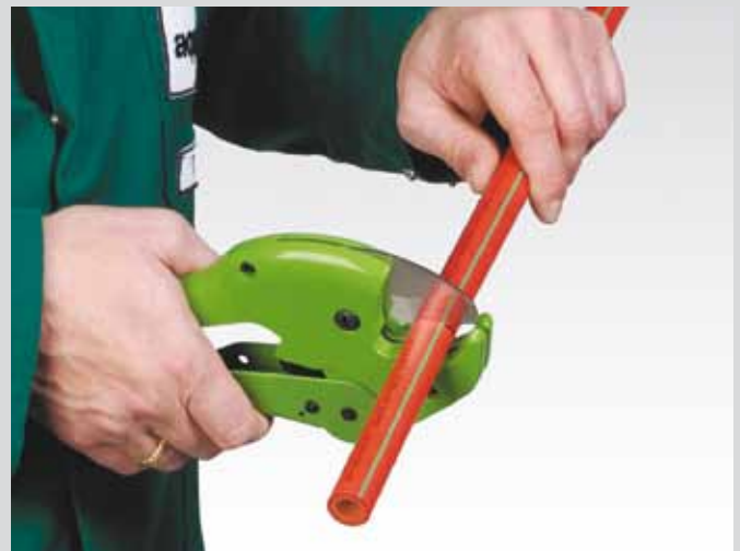
Cutting of the pipe
