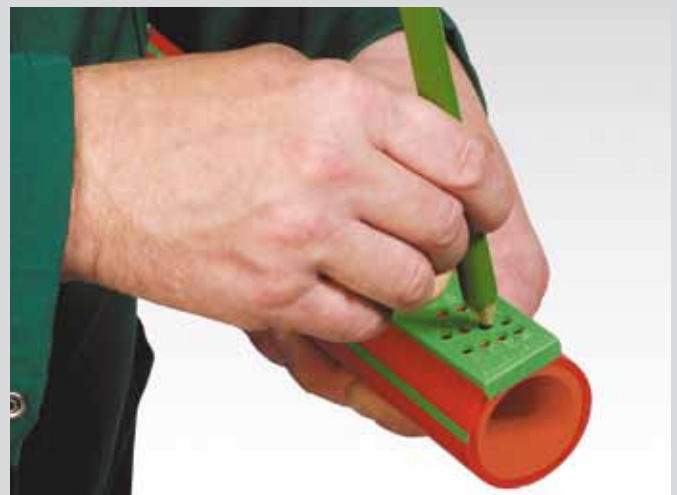
Marking of the welding depth
