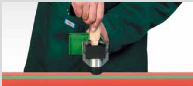
Heat-up of pipe...
