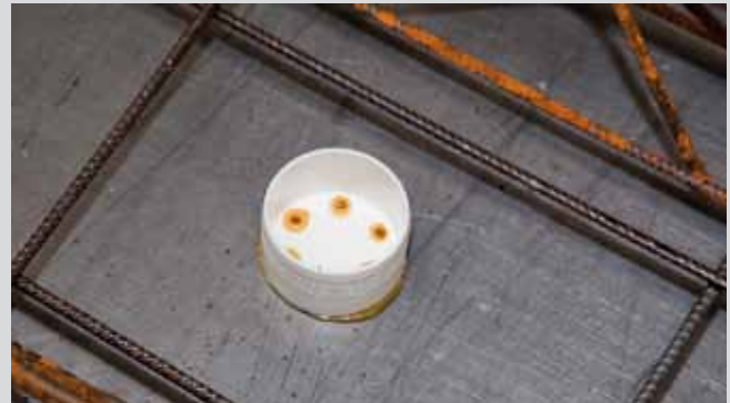
Base part of sprinkler outlet Art.-No. 4114190 for concealed sprinklers. Attachment with hot-melt adhesive.
