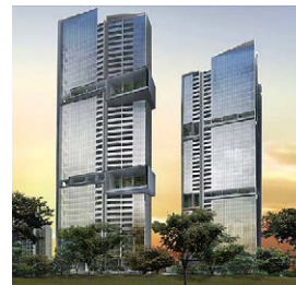
Echelon Tower Singapore Construction period: 2013–2016
