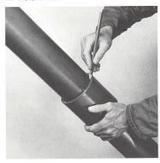
Then clean thoroughly with Tangit Cleanser H. Spray Tangit Cleanser H onto a piece of soft paper, e.g. tissue paper, and thoroughly clean the mating surfaces of all grease and dirt. Use a new piece of tissue paper for each cleaning operation. Any ice should be removed by careful heating.
