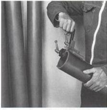
First clean the mating surface (outside of pipe end, inside of socket). Then mark the insertion depth on the end of the pipe to enable application of the necessary adhesive and full depth insertion of the pipe to be checked. With conical fittings, measure the length to be bonded and mark pipe end.
