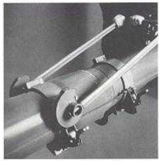
For dimensions exceeding DN 80, two people should work simultaneously on applying the cement to the pipe and socket.
