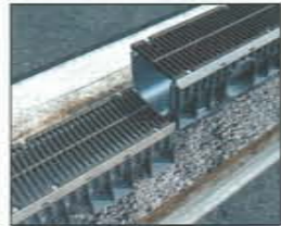
Setting the channel, haunching and filling in
