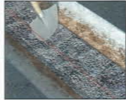
Setting the channel, haunching and filling in
