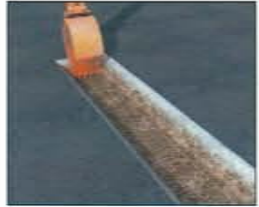
Setting the channel, haunching and filling in
