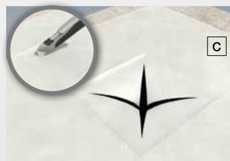
Use a safety cutter to cut the central area into a cross
