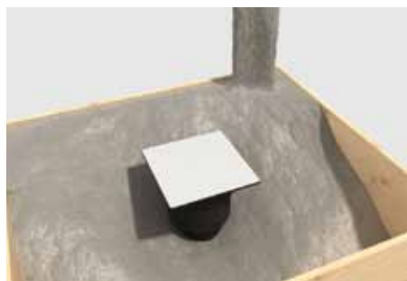
Pour the concrete slab or plug with an anchoring mortar. The polystyrene protector is flush with the poured surface.
